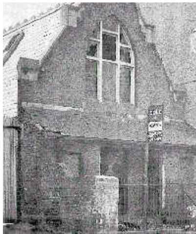
Derelict Church Hall which became the De Laune Clubroom
